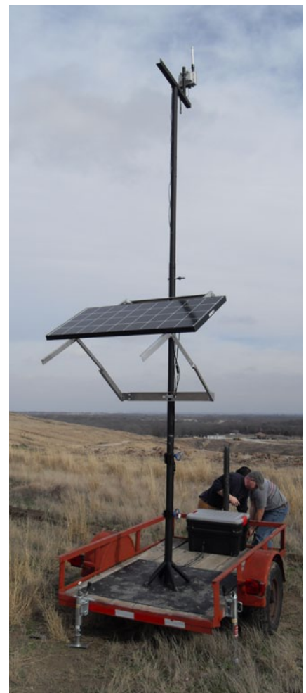
Repeater station undergoing installation.
